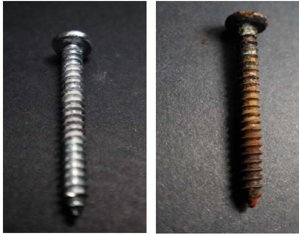
Figure 4-21- Comparison of corrosion of zinc coated fasteners in MgO board F (steel) (left) and MgO board B (steel) (right)
